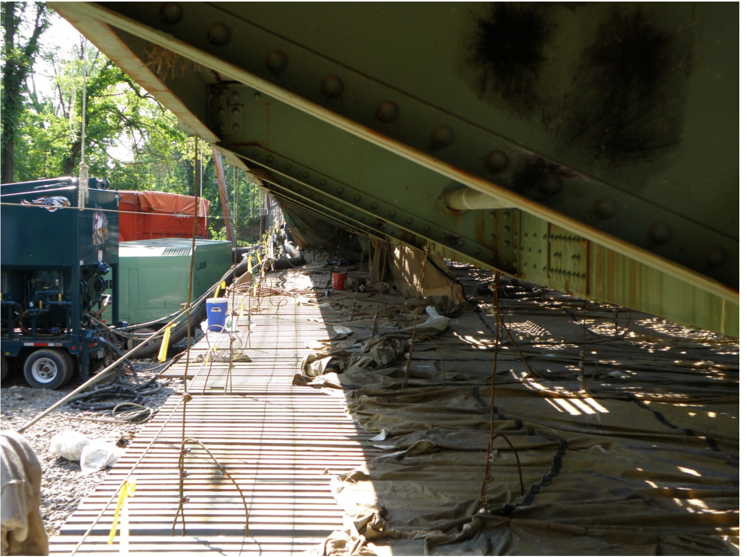
Lower Level Cable/Metal Deck Platform
