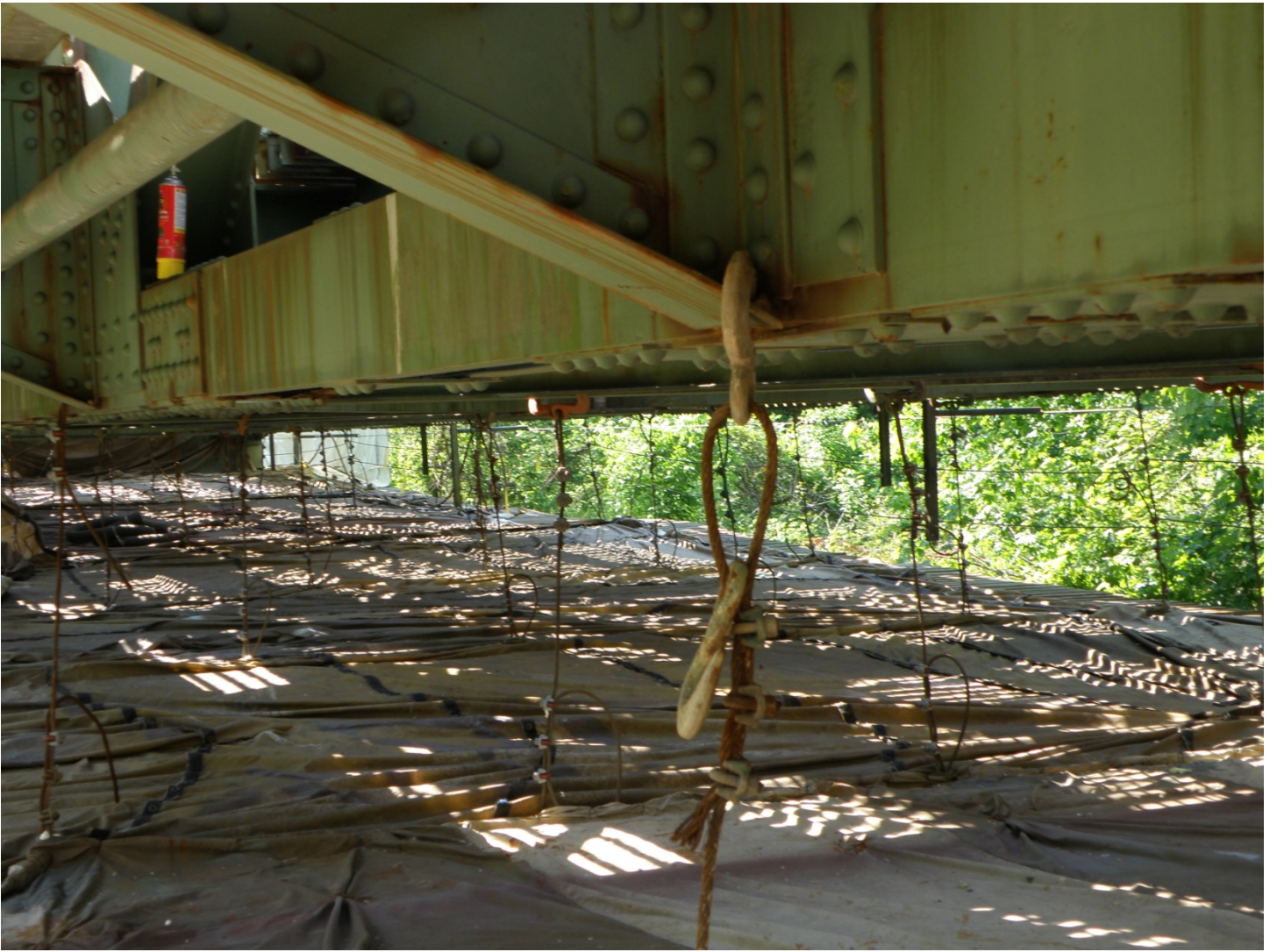
Lower Level Cable/Metal Deck Platform
