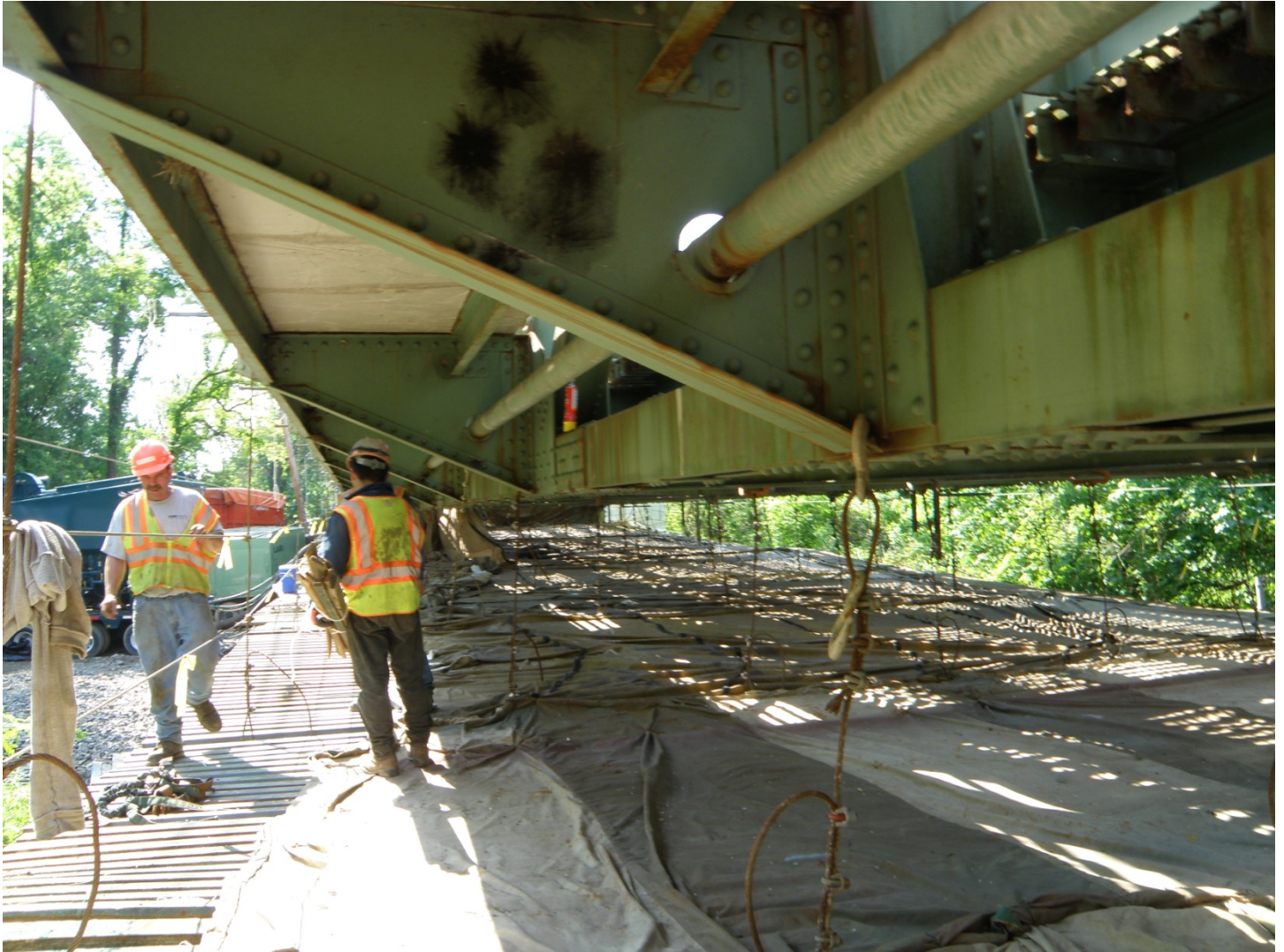
Lower Level Cable/Metal Deck Platform
